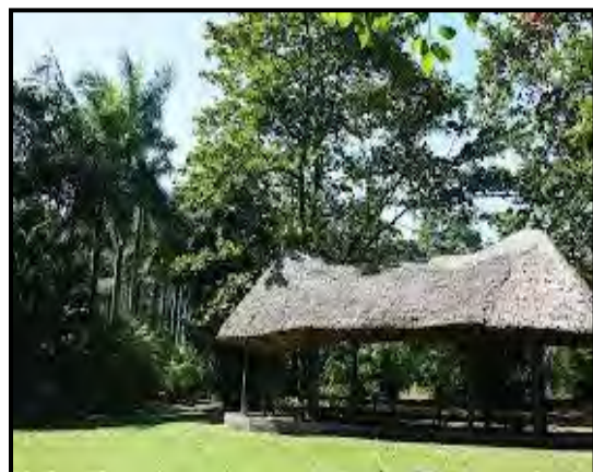
Rest house made from kunjai
