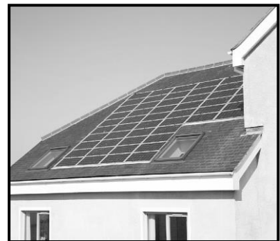
House water is heated by solar energy
