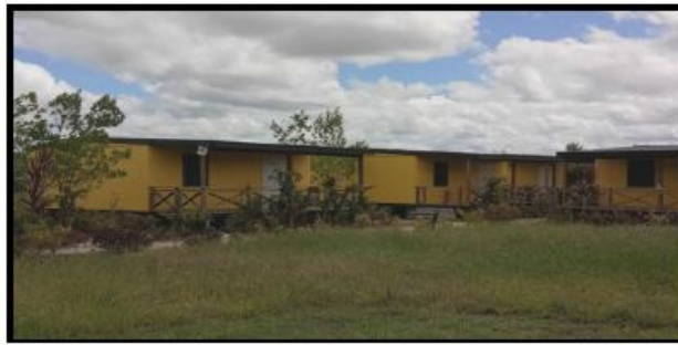
Outside view of the classrooms
