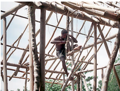
Figure 1: House building, East Sepik
