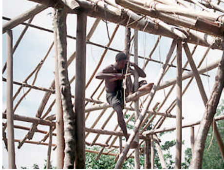
Figure 1: House building, East Sepik
