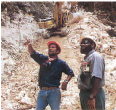
Excavating for mine infrastructure
