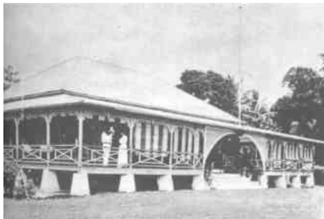
Gunantambu – Emma's house at Ralum, near Kokopo (1913). The house was destroyed during the Japanese occupation 1942-45. (from Queen Emma)
