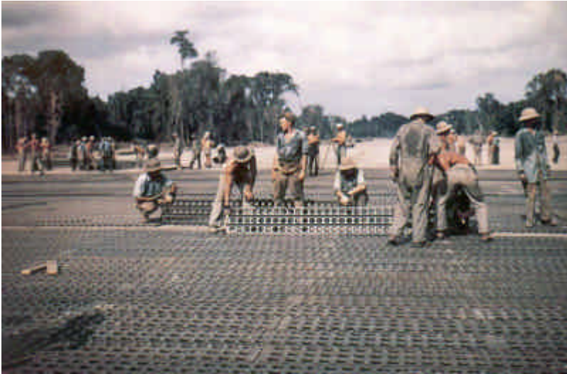
Seabees laying steel mats during the construction of an airfield on Bougainville in December 1943. These mats were known as Marsden mats and remnants can still be found throughout PNG (from 'World War II in the Pacific').
