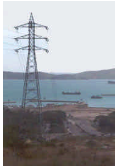
Figure 1: High voltage power supply lines. Source: N. Lauer.
