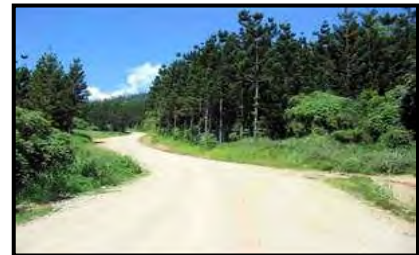
Road built through the forest
