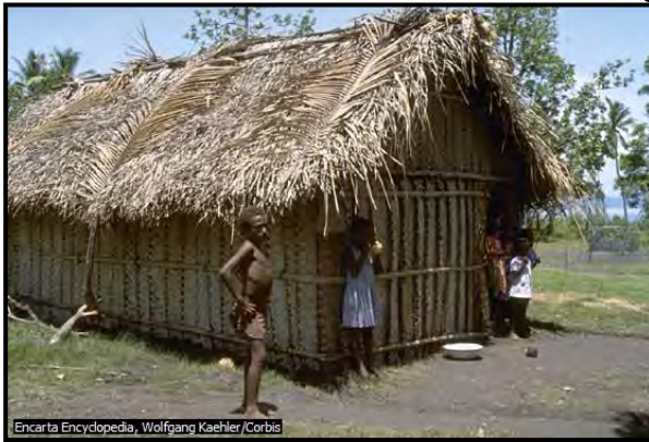
Thatched roof home
