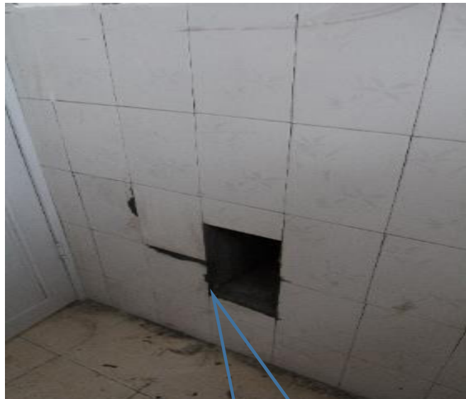
A hole connect private room and incinerator (Fire Box)
