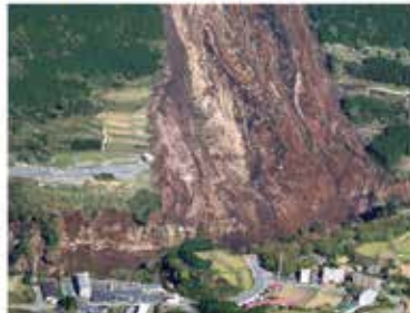
Parts of a mountain and a town destroyed by landslide.
