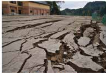
Earthquakes cause cracks on the ground.
